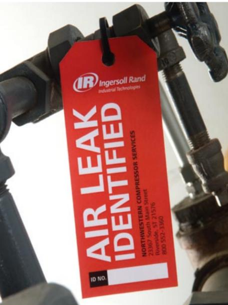
Our durable leak assessment tags are designed to remain in place for years, so we can make sure the leak was repaired correctly when we return for your optional annual checkup. Tags available in beige or red with calendar on the back to track, ID, repair and verify.
